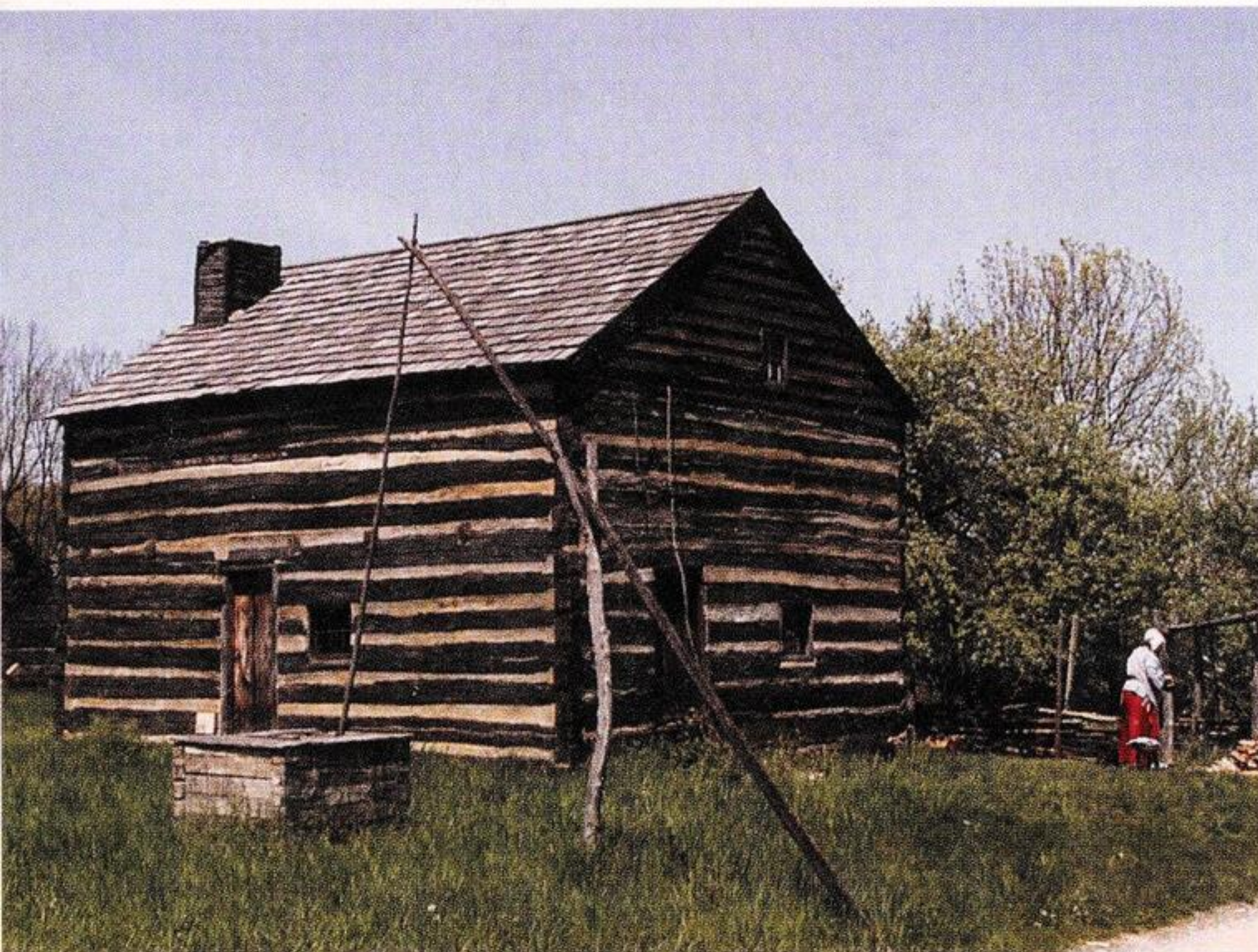
This log cabin is typical of ones built in New York in Caroline's time. You can see it today at Genesee Country Village and Museum in Mumford, New York.
