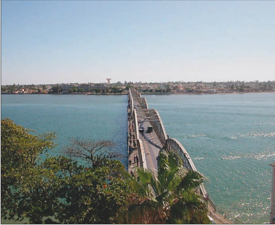
The Faidherbe Bridge crosses the Senegal River at Saint-Louis. The bridge was named for the former governor of French Senegal, Commander Louis Faidherbe.
