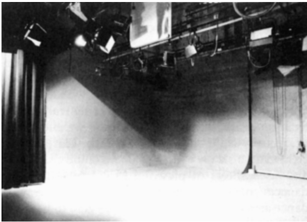
Figure 2.6 This hard cyc is in the corner of the studio. The picture shows how it is built to merge with the floor. The curtain on the left of the picture is drawn around in front of the hard cyc to create a soft cyc.
