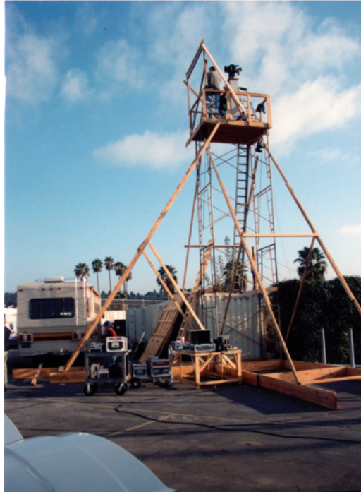
Figure 2.6: In some cases it was necessary to build steady platforms for the camera. This structure built by master grip Larry Shuler shows the typical opposing strut design that takes all movement out of the tower. Courtesy of Illusion Arts.
