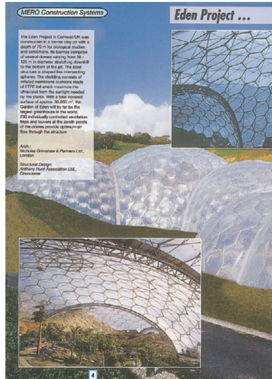
Plate 24 Eden Project, Cornwall, UK, MERO construction system, architects: Nicholas Grimshaw and Partners, structural design: Anthony Hunt Association Ltd. Several spherical domes varying from 38 to 125 m in diameter, double-layer structure of hollow profiles, hexagonal geometry, bolted connections. © MERO.
