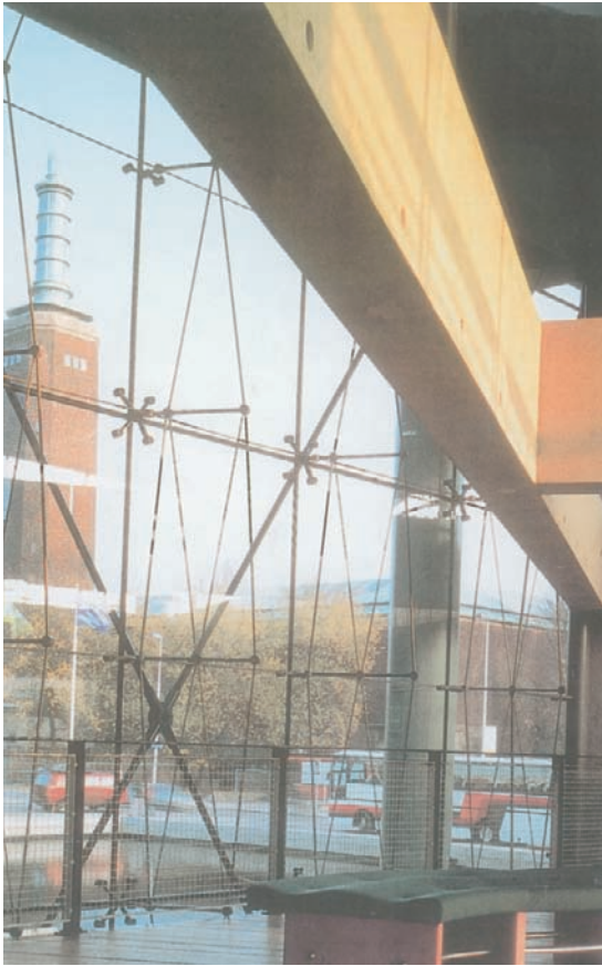
Plate 19 Netherlands Architecture Institute, Rotterdam, The Netherlands, 1988–93, architect: Jo Coenen. Structural glass façade.
