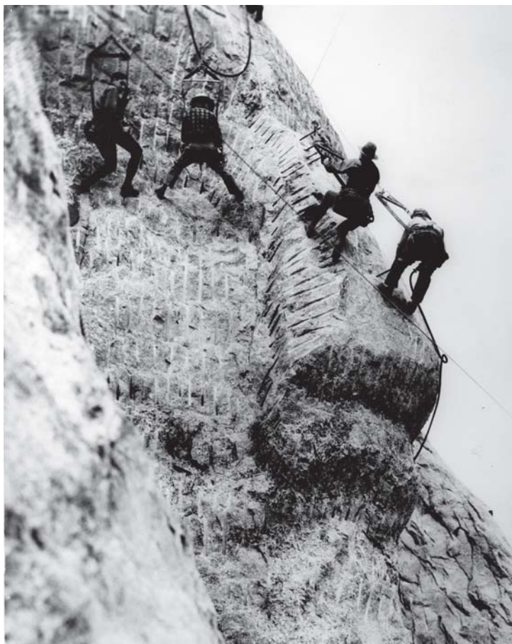
18. Workers on Mount Rushmore fashioning Washington's nose and lips with compressed air drills. Photo courtesy of the State Archives of the South Dakota State Historical Society.
