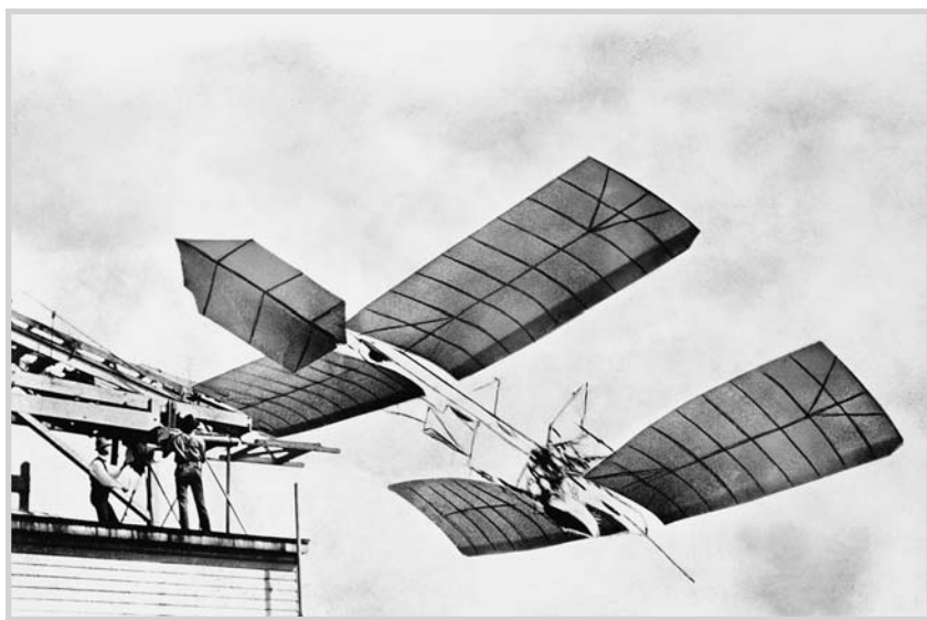
Launched from a houseboat in October and again in December 1903, the Langley Aerodrome A twice plunged into the Potomac River instead of flying.
