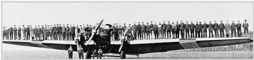
Junkers employees demonstrate the strength of the Junkers G.23's fully cantilevered wing in 1924.
