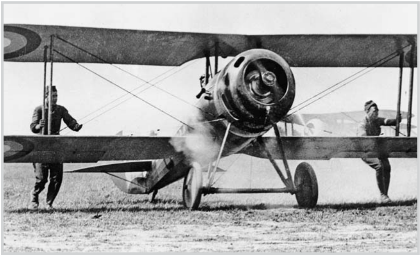
A Gnome rotary engine spins together with its propeller in this Nieuport 28 as it prepares for takeoff in World War I.
