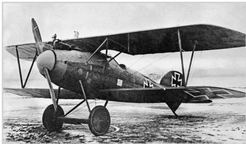
The Albatros D.Va was one of several German World War I fighter planes with a molded-plywood fuselage.
