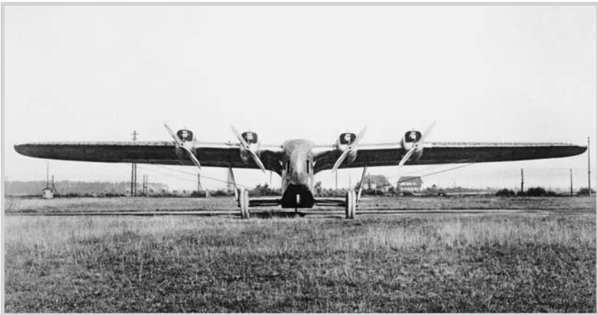
The Zeppelin-Staaken E.4250 of 1920 might have hastened the adoption of all-metal, stressed-skin construction had it not been ordered destroyed under the terms of the Versailles Treaty.
