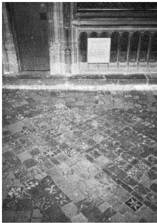
Figure 12.2 Conserved tiles, many of which are in situ, completed in the first stage of work. Isolated replica tiles are visible (Photograph, Peter Bird)
