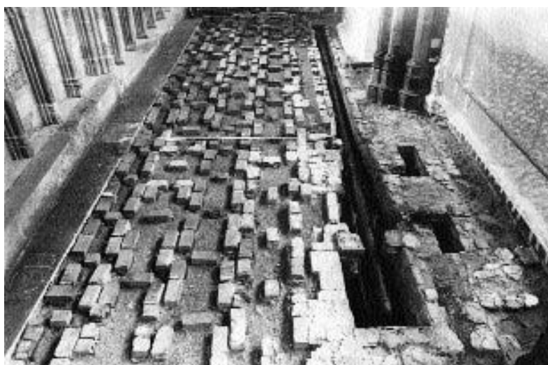
Figure 2.2 Lichfield Cathedral. Unusual brick sub-structure to support Scott's limestone paving of 1860 in the north choir aisle (Photograph, Warwick Rodwell)
