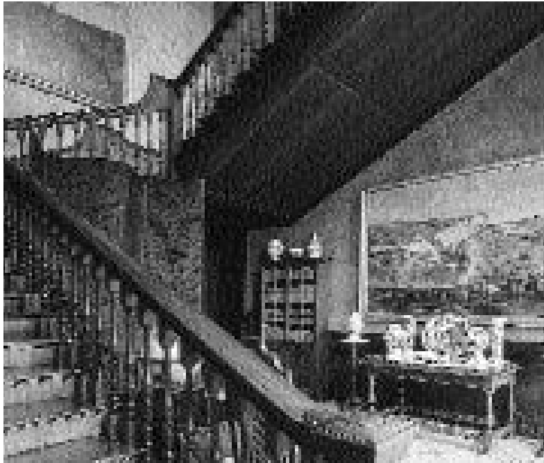
Plate 73 At Dyrham Park, near Bath, this main staircase cannot bear the weight of the constant flow of visitors. The treads and the landing also show damage from sharp heels. Now closed to the public – see page 198 (Photograph, National Trust)
