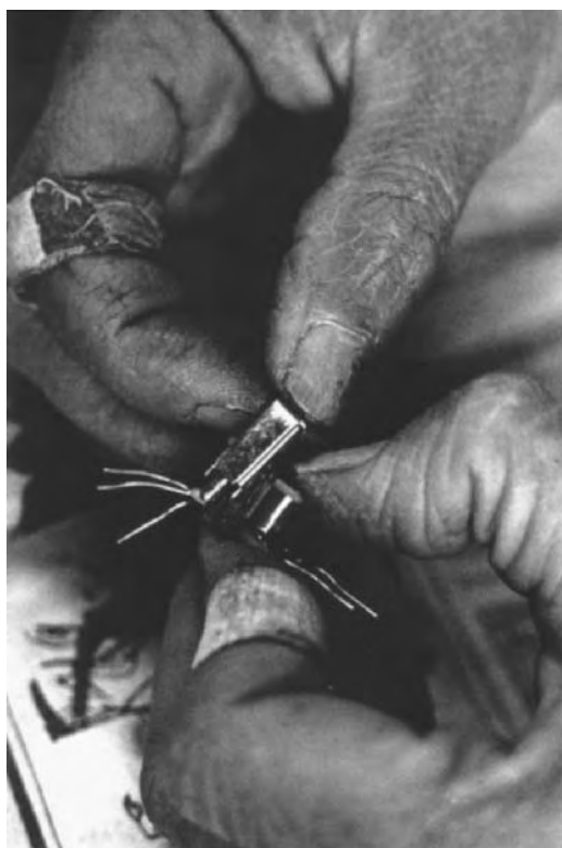
Figure 6.6 The hands qua transistor assembling machine. Hanabusa Shinzō, "Rural Electronics Manufacturing, Ina City, Nagano Prefecture" (Nōson denshi kōgyō), 1964. © Hanabusa Shinzō.
