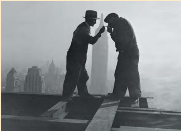
Rockefeller Center construction workers, 1932
