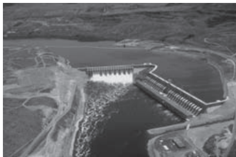
A run-of-the-river hydroelectric plant
