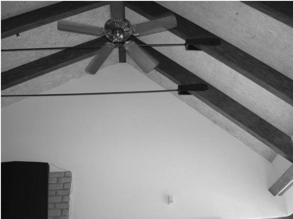
Figure 7.3 Exposed beam ceiling inside of 45° slope roof.
