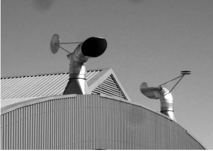
Unidirectional windcatchers can be striking architectural features (Reproduced with permission from Arup – Mike Rainbow)
