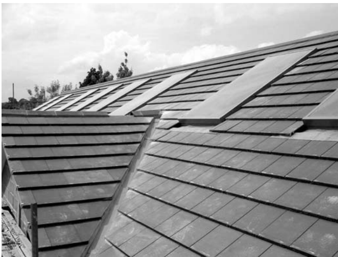
Roof-mounted thermosyphoning air panels can be unobtrusive (Reproduced with permission from Nuaire)
