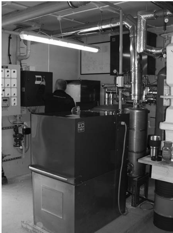
Natural gas fuelled CHP, like this 15kW installation from EC Power, is a well-developed technology (Reproduced with permission from EC Power)
