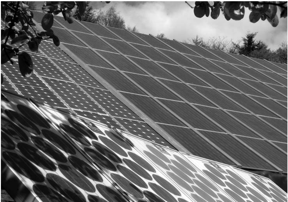
Monocrystalline and polycrystalline solar PV panels at the Centre for Alternative Technology Wales (Reproduced with permission from Centre for Advanced Technology)
