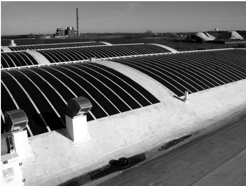
Roofing membranes incorporating PV cells open up new possibilities (Reproduced with permission from United Solar Ovonics)
