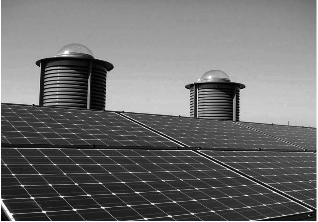
This roof features solar PV, windcatchers and lightpipes (Reproduced with permission from Monodraught)
