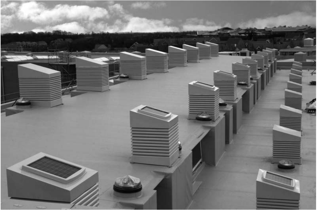
Solar PV-powered fan-boosted windcatchers (Reproduced with permission from Monodraught)
