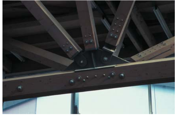
▲ 7.24 Web members connect to a truss bottom-chord.
