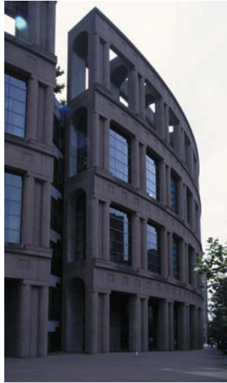
▲ 4.15 Library Square, Vancouver, Canada, Moshe Safdie and Associates Inc., 1995. A gap reveals the cross-section of the screening frame and a glimpse of the main library block behind.
