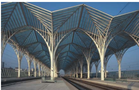
▲ 9.4 A view along the canopy structure.
