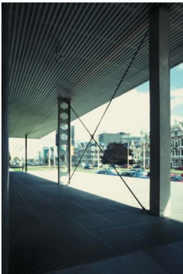
▲ 7.11 Two of the three differently detailed columns.
