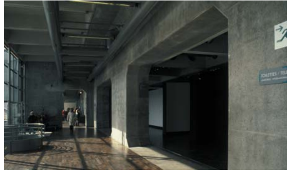
▲ 3.19 An interior vierendeel truss to the right.
