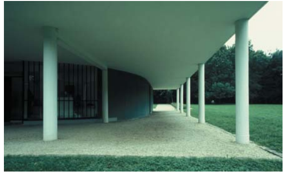
▲ 7.65 Plain exterior column and beam detailing.
