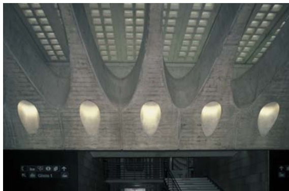
▲ 8.12 Stadelhofen Railway Station, Zürich, Switzerland, Santiago Calatrava, 1990. Integration of structure and artificial lighting.
