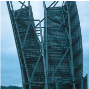
▲ 7.20 The tower structure.
