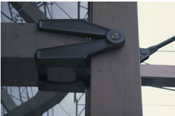
▲ 7.31 A beam-column connection where a horizontal gap between the castings allows for a down-pipe to pass through the detail where required.
