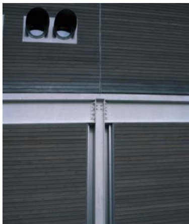
▲ 2.5 Exterior column recessed within an external wall.
