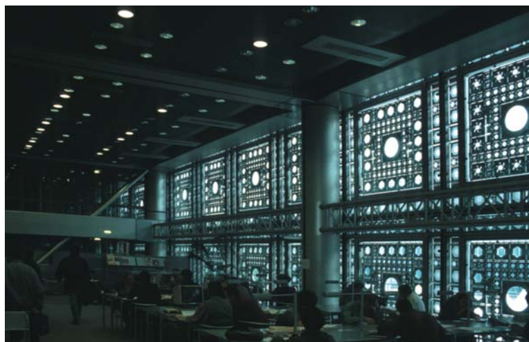
▲ 7.55 Internal horizontal trusses in the library.
