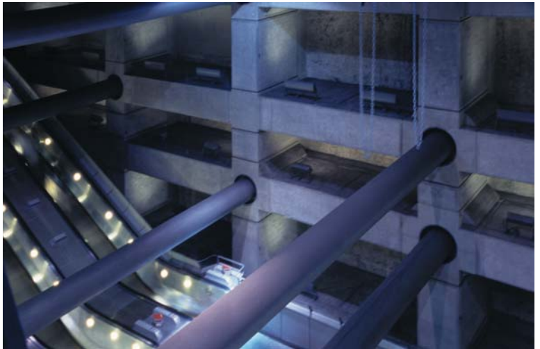
▲ 6.33 Horizontal props between side walls.
