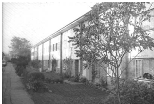
Figure 8.28 Harlow, housing and landscape
