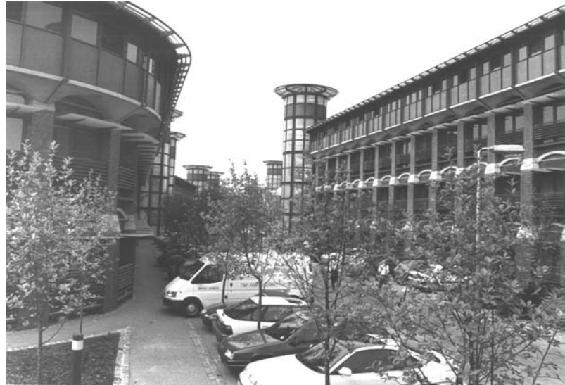
Figure 9.39 Inland Revenue Building, Nottingham
