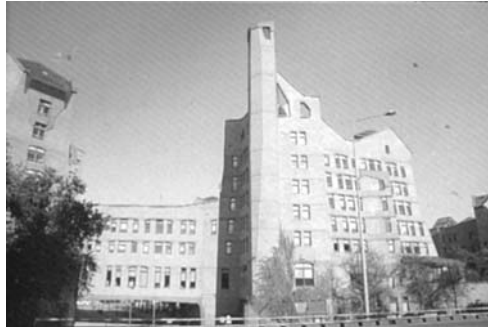
Figure 2.20 NMB Bank Headquarters, Amsterdam
