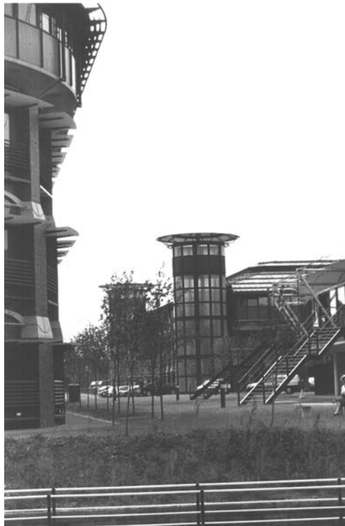
Figure 9.38 Inland Revenue Building, Nottingham
