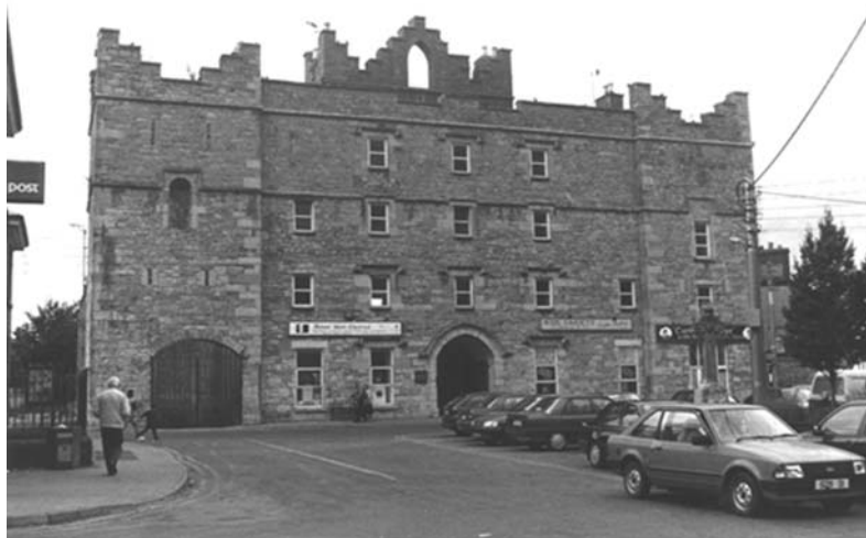
Figure 6.18 Roscommon, Ireland: former jail
