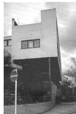
Figure 6.28 Building by Le Corbusier, Stuttgart
