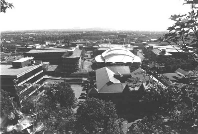
Figure 9.37 Inland Revenue Building, Nottingham
