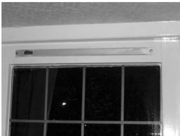
Figure 5.1 Trickle ventilator
