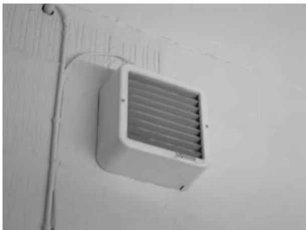
Figure 5.8 Typical domestic extract fan
